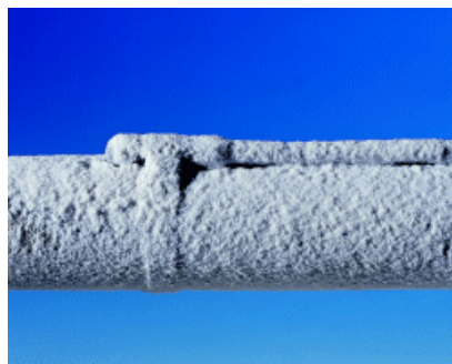
Temperature measurement of frosted pipelines
