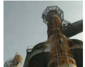
EP Exit Chimney
